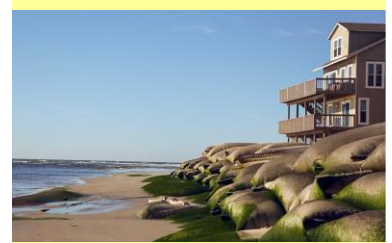
Because of beach erosion, officials on Topsail Island, N.C., have had to combat the rising water with large sandbags. Credit Logan R. Cyrus for The New York Times
